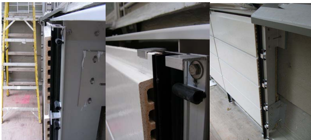
Photos shows sill horizontal channel with sill part installed with tiles
