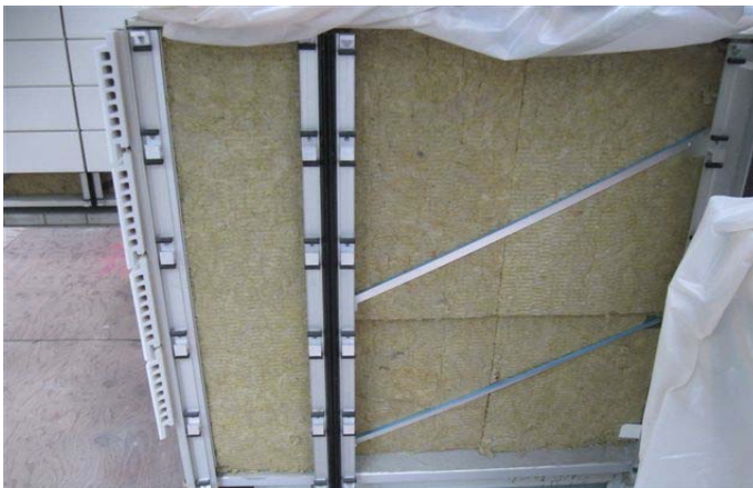
Photos shows insulation batts retained via aluminium angles
