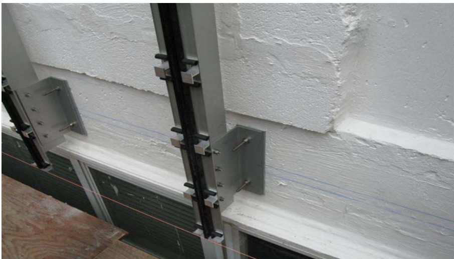
Photo shows brackets installed with vertical tracks attached (note string line)
